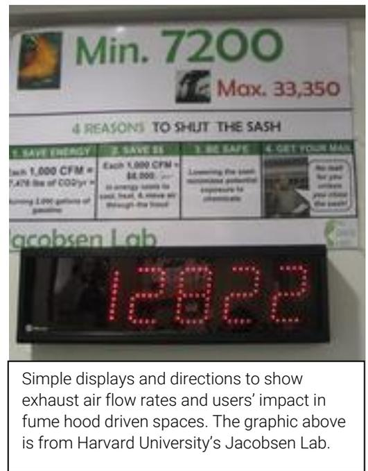
Simple displays and directions to show exhaust air flow rates and users’ impact in fume hood driven spaces. The graphic above is from Harvard University’s Jacobsen Lab.
